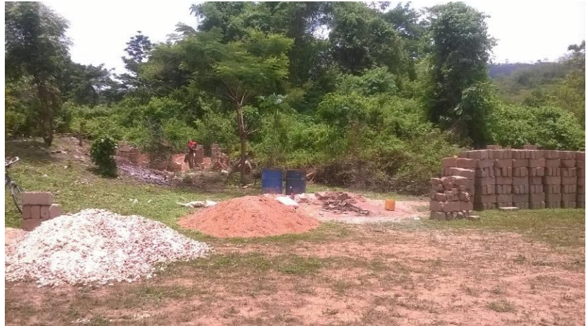
Site layout with blocks stacked for construction of the walls.
