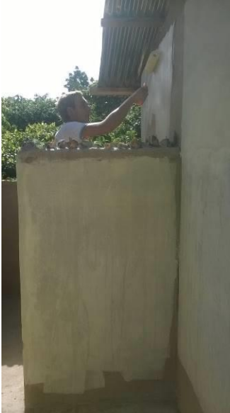
Final paint and finishing touches.
