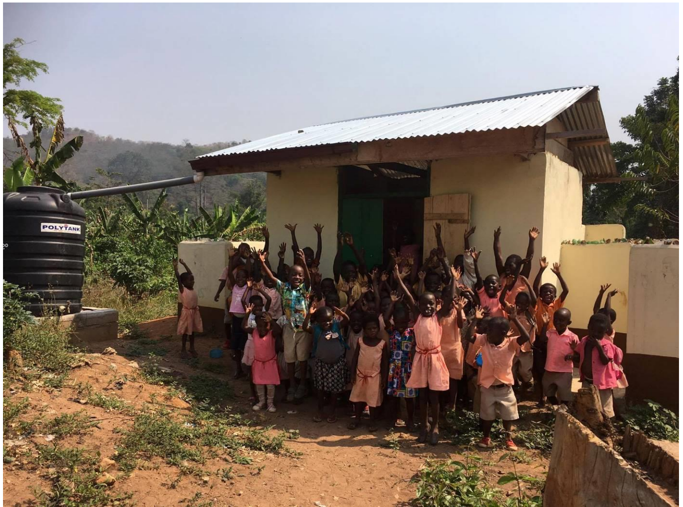
Completed toilet block with water tank in place.
