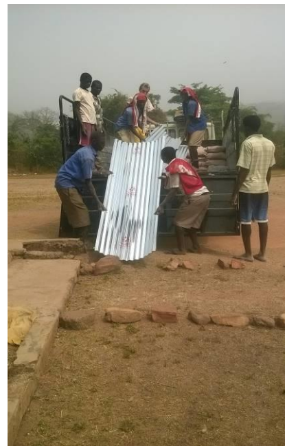
Sheet material for the roofs being delivered
