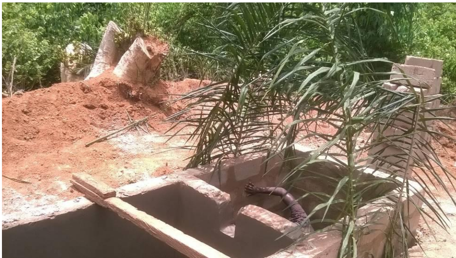
The underground tanks were rendered to make them watertight.
