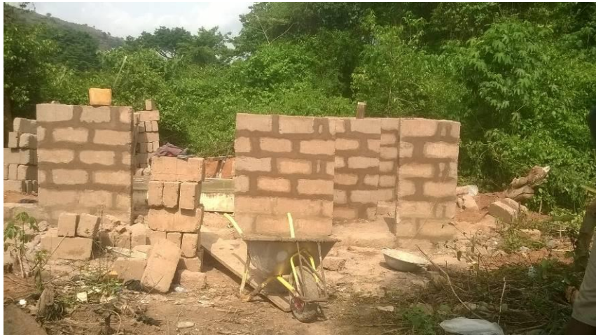
Wall construction underway.
